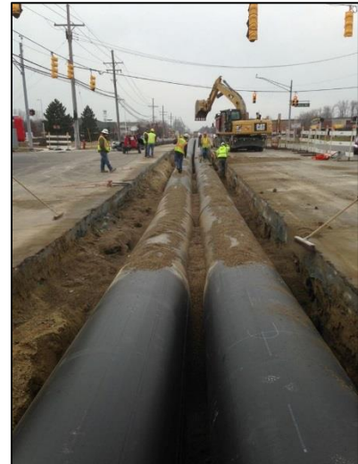
Long-term bypass pipes are installed at 15 Mile and Utica roads.
