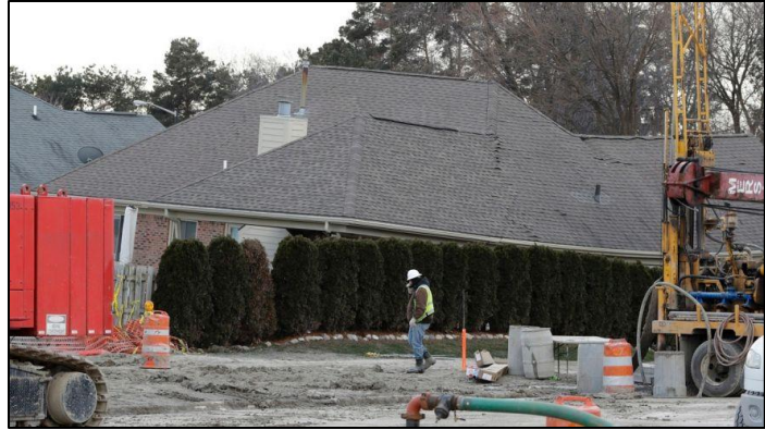
Damaged home on Eberlein Drive (seen from 15 Mile Road).
